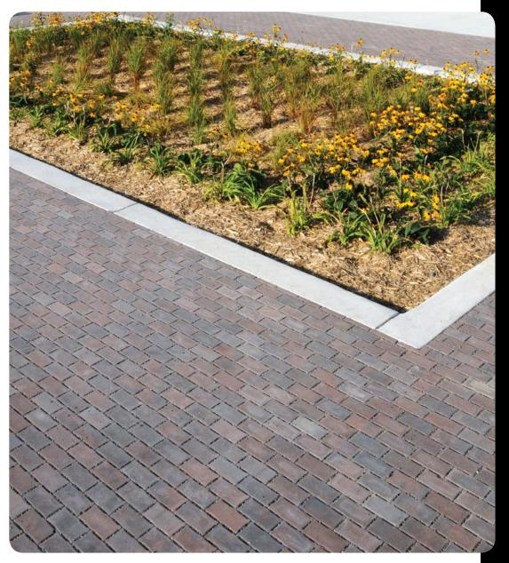
Willow Creek permeable pavers are helping manage stormwater runoff at Century College in White Bear Lake, MN. To minimize runoff, the 16-acre site employs about 4,000 square feet of Willow Creek Brickstone Permeable pavers, plus porous asphalt and concrete. The surfaces direct runoff to rain gardens through which it infiltrates to underground storage chambers.
